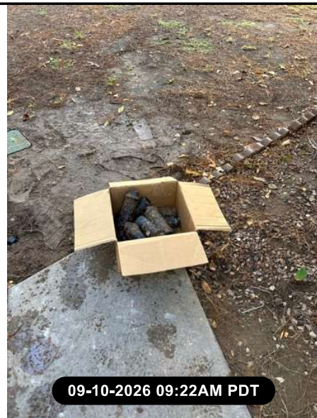
Old sprinklers replaced
