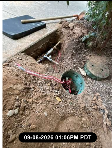
Wires preparation for Wire Ride
